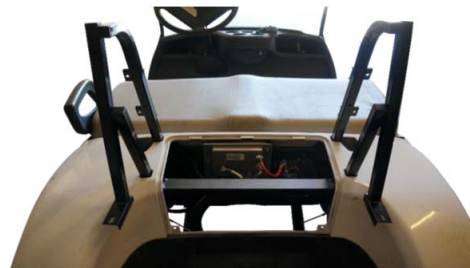
Step 2: Install main brackets on cart using original factory hardware.
