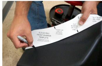
3. Using a marking tool, trace the template onto the bumper on the line that reads "CUT BUMPER ON THIS LINE".
